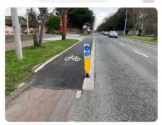
Figure 4-60: Transition from carriageway to cycle track
